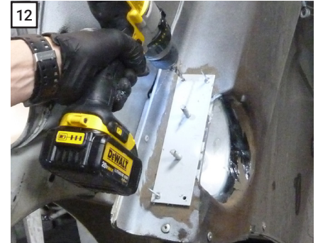
12 With a rivet temporarily placed in the first hole as a guide, drill the remaining rivet holes. Remove the plate, bolts, and rivet.
