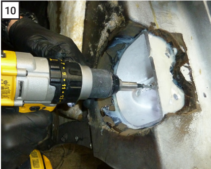
10 Install the plug & use a #10 wood screw to secure the plug in position. Wipe up excess adhesive with a gloved finger or spreader.
