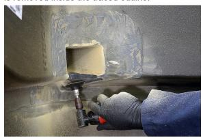
5. THOROUGHLY <u>HAND SAND</u> the inside of the pockets anywhere the Roloc<sup>™</sup> disc couldn't reach with 60 grit or coarser sandpaper, make sure all paint is removed and the area is thoroughly roughened. Roughen all remaining surfaces to be bonded with 60 grit or coarser sandpaper.
