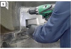
Using a permanent marker or a drill, mark the hole locations for the screws. (Marking with a drill, shown.)
