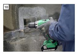
Drill all seven (7) hole locations and remove the dust using compressed air or a cloth dampened with EcoPrep plastic cleaner. Make sure the area is <u>completely</u> dry before proceeding.
