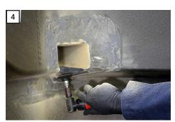
Grind the area where the casting will be bonded with a 50 grit or coarser Roloc™ disc. Be sure all paint is removed inside the traced outline.
