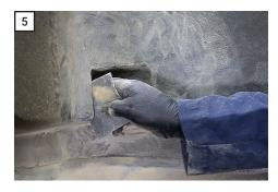
THOROUGHLY <u>HAND SAND</u> the inside of the pockets anywhere the Roloc™ disc couldn't reach with 60 grit or coarser sandpaper, make sure all paint is removed and the area is thoroughly roughened. Roughen all remaining surfaces to be bonded with 60 grit or coarser sandpaper.
