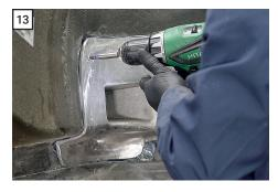
Install the casting and secure it into position loosely with the included screws. DO NOT TIGHTEN the screws until all screws are in place and the casting is seated into the pocket correctly. Hand tighten the screws only until firmly snug. If the screws are installed too tightly, too much adhesive will squeeze out, starving the joint and weakening the bond.
