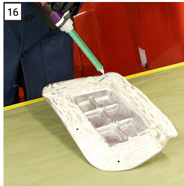
16 Apply the other half of the 2510 PlastiFix adhesive to the mating surface of the casting.
